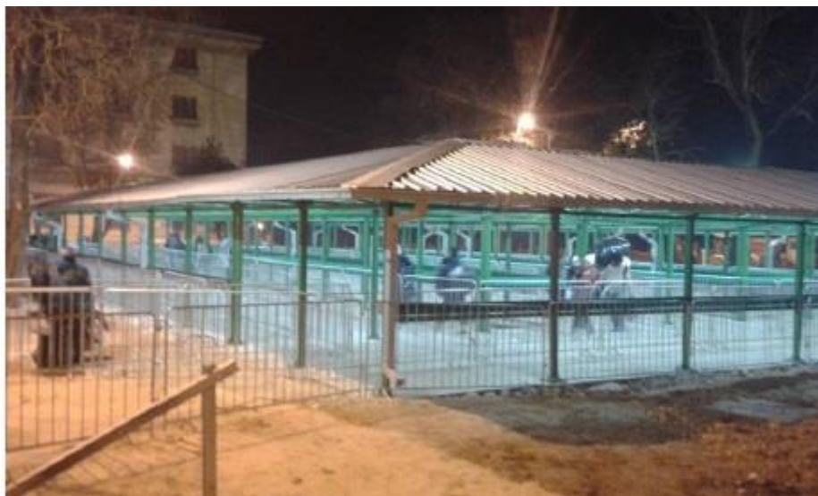
Picture 2 Improved conditions for the reception of refugees/ migrants in the Reception Centre in Preševo – a hood set on the entrance of the Reception Centre
